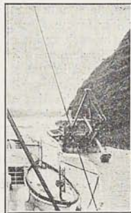
Dredge Working in Culebra Cut
